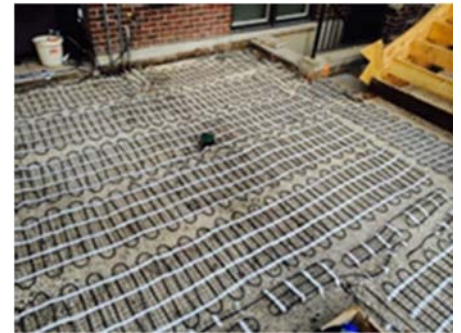
Gutter & Roof Installation- Melts Snow/Ice to Prevent Ice Damming and Water Damage
